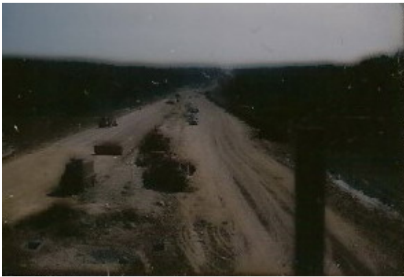
Massachusetts Turnpike under construction in 1956
